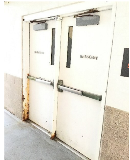
Photo A5 – Main And Upper Concourse Typical Fire Rated Door Assembly.
