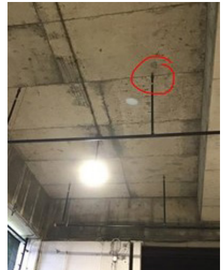
Photo FP4 – Services Drive Sprinkler Deflector Clearance
