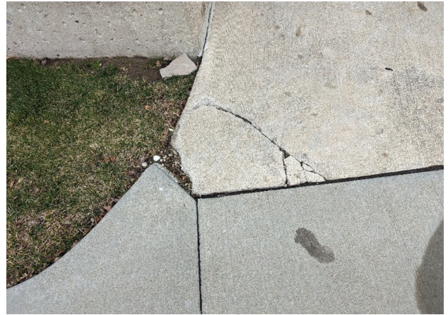
Photo C1 – Typical Cracked Concrete
