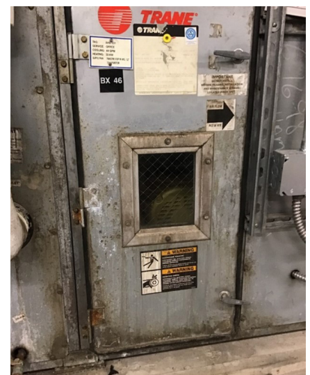
Photo M2 – Ahu Deterioration
