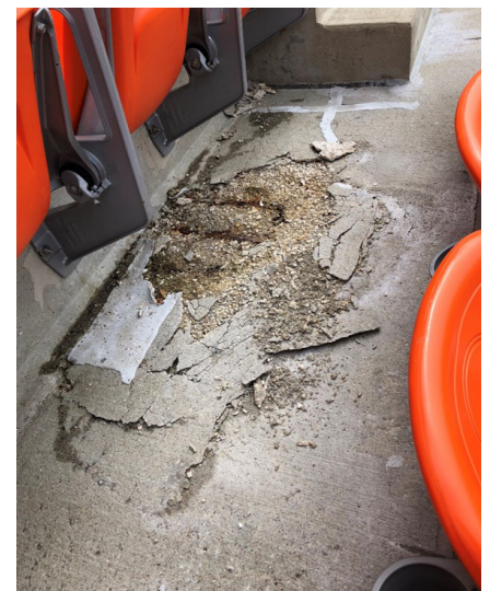
Photo S1 – Typical Spalled Concrete
