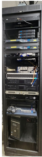
Photos B17 – Modulators, Satellite Receivers and Trunk Amplifier
