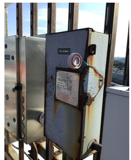
Photo E2 – Field Light Disconnect
