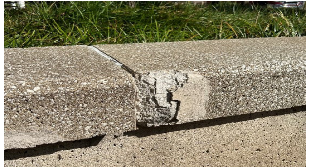
Photo L5 – Planter Bed Precast Concrete Coping In Poor Condition
