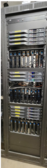
Photos B19 – Modulators, Satellite Receivers and Trunk Amplifier
