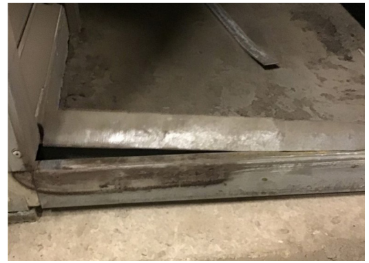
Photo M3 – Edge And Door Seals Worn On Ahu Access Door.
