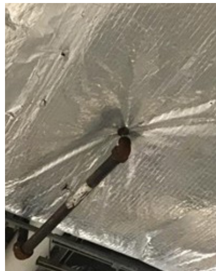
Photo FP3 – Duct Insulation Sagging Interfering With Sprinkler Deflector Clearance.
