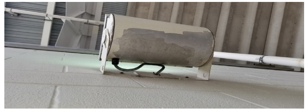
Photo E8 - Typical Wall Mounted Hid Fixture Showing Corrosion.
