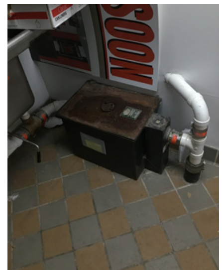
Photo P4 – Rotted grease trap
