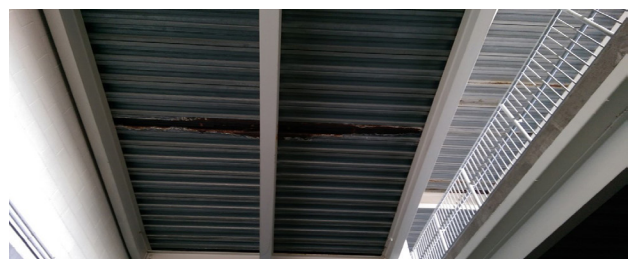
Photo S8 – Typical Corroded Metal Floor Deck at Ramps
