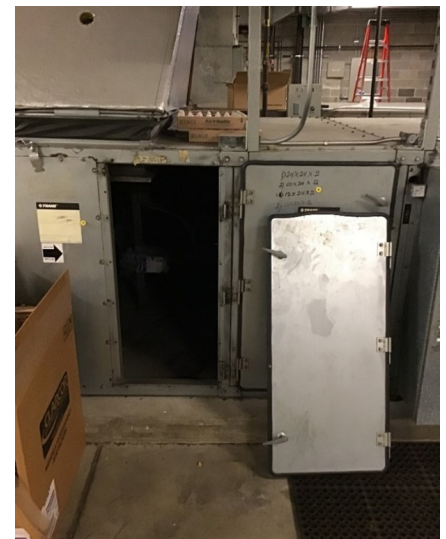
Photo M1 – Door Off The Hinges On Ahu
