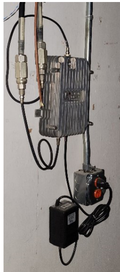
Photos B20 – Modulators, Satellite Receivers and Trunk Amplifier
