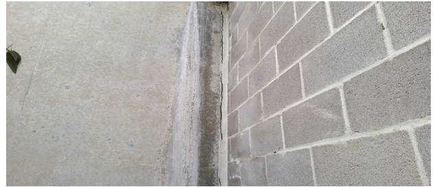
Photo S6 – Typical Failed Backer Rod & Sealant Joint
