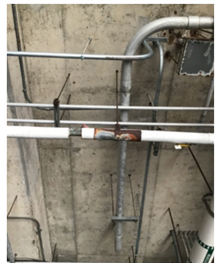
Photo P2 – Deteriorating pipe hangers
