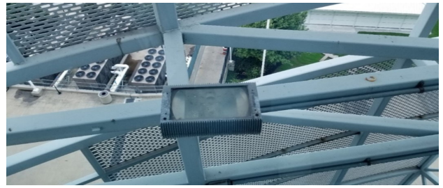
Photo E5 - Hid Fixture Mounted Behind Windscreen
