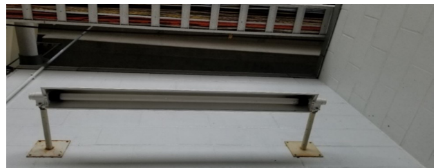
Photo E4 - Linear Fluorescent Fixture Mounted In Concourse.
