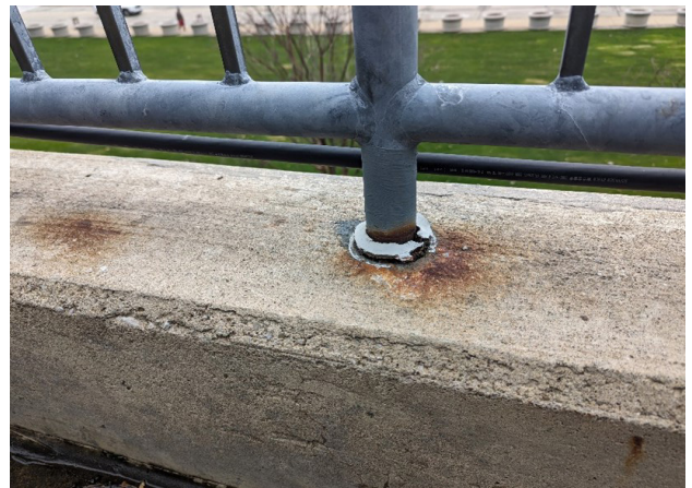
Photo C2 – Typical Failed Sealant at Guardrail Post
