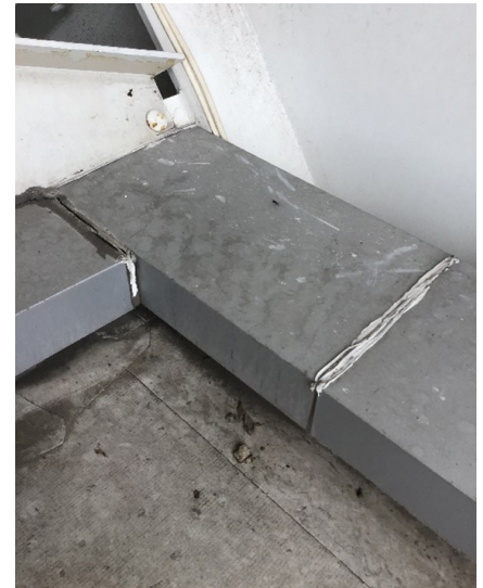
Photo A1 – Sealant Joints At Roof Parapet Cap.
