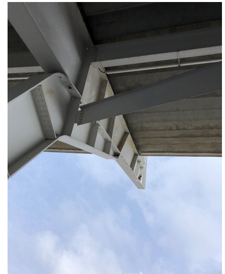
Photo S9 – Typical Surface Corrosion on Structural Framing Member
