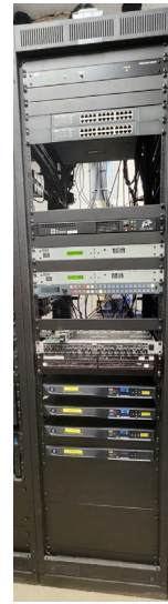
Photos B18 – Modulators, Satellite Receivers and Trunk Amplifier
