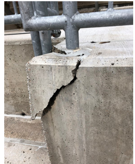
Photo S3 – Typical Concrete Damage at Guard Rail Post
