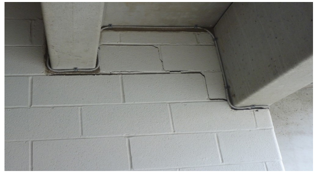
Photo S5 – Typical Masonry Cracking at Vomitory Wall
