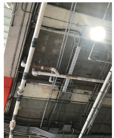
Photo P3 – Deteriorated storm pipe insulation
