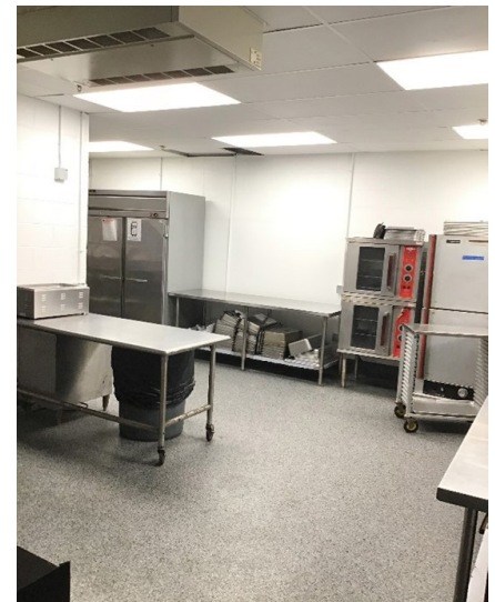
Photo A11 – Epoxy Floor In Kitchen Areas
