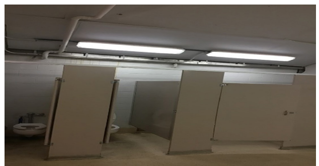
Photo E12 - Typical Toilet Room Wall Mounted Fluorescent Fixture.
