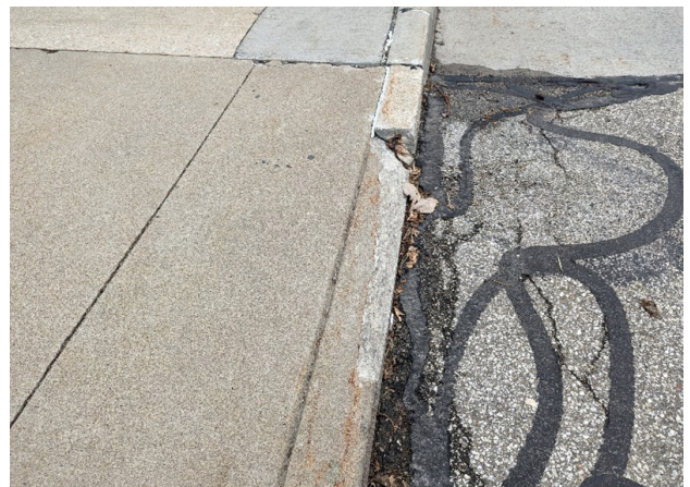
Photo C3 – Typical Failed Curb
